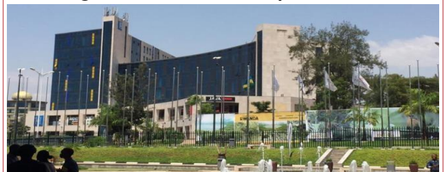
The completed Kigali Heights
